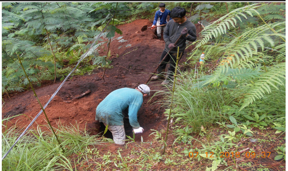
HUMAN-MADE CHANGES. Baguio Water District has set its eye to take advantage of the massive amount of rain it gets annually. In this file photo, personnel are constructing ditches within Busol watershed to catch and trap runoff water therefore, accelerating the recharging of underground water sources to meet the daily water demands of the City.
